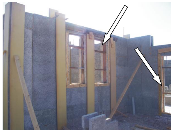
Bracing of long straight runs.
